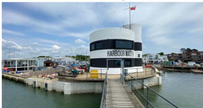
The completed works at the Harbour Master's Office
