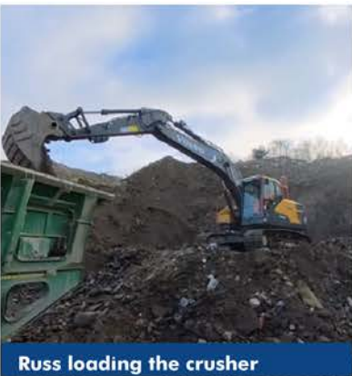
Russ loading the crusher
