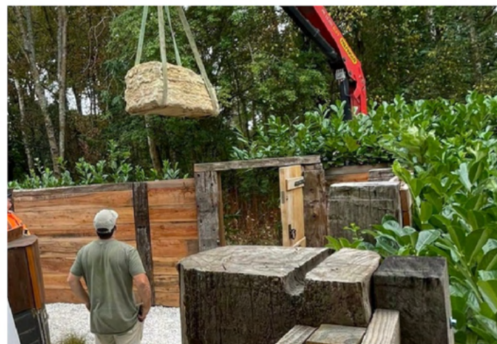
Tim delivering the boulders to site
