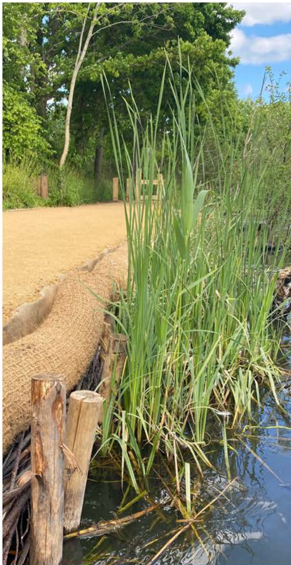
The edge of the new pathways finished with the coir rolls
