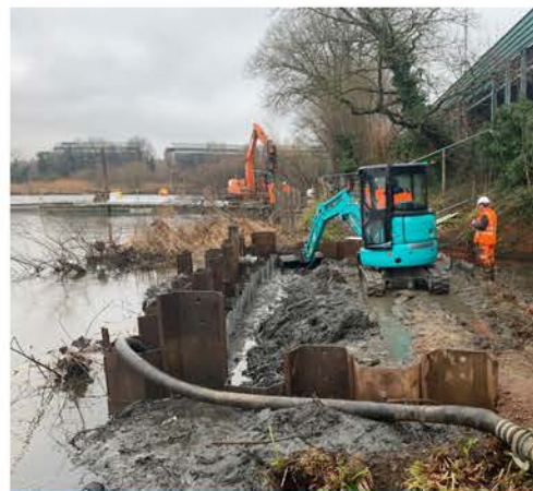
The sheet pile structures used to improve the pathways
