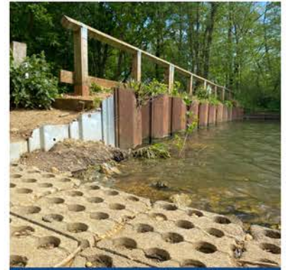
The new Slipway at Boat House Corner
