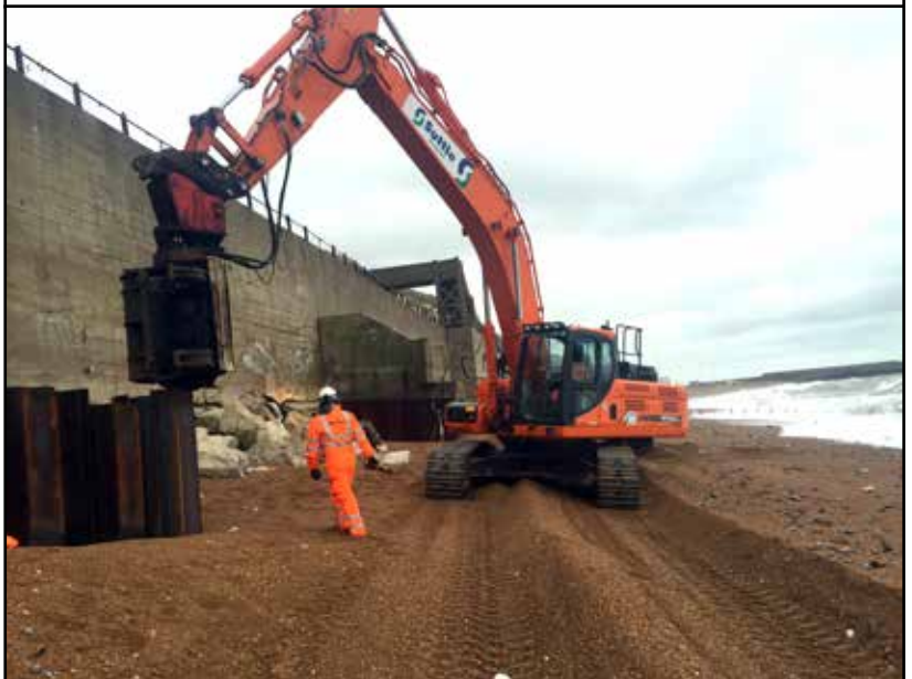
Team effort: Suttles staff worked through Christmas to reinforce damaged coastal defences at Dover. Below: piling is moved into place
