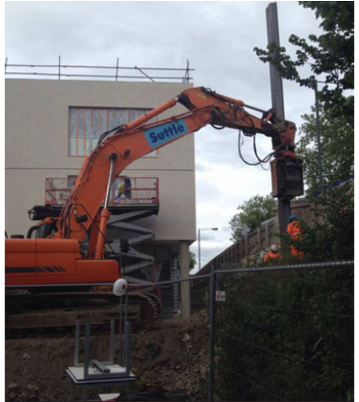
(L-R) 11m PU28 piles were installed by a Movax SP70F4 at Bexley College
