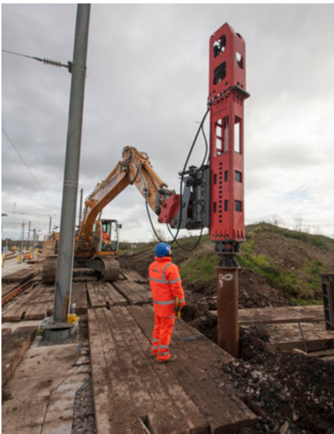
(L-R) Our Movax DH20 was used to drive in piles at the Hitachi train service depot at Stoke Gifford
