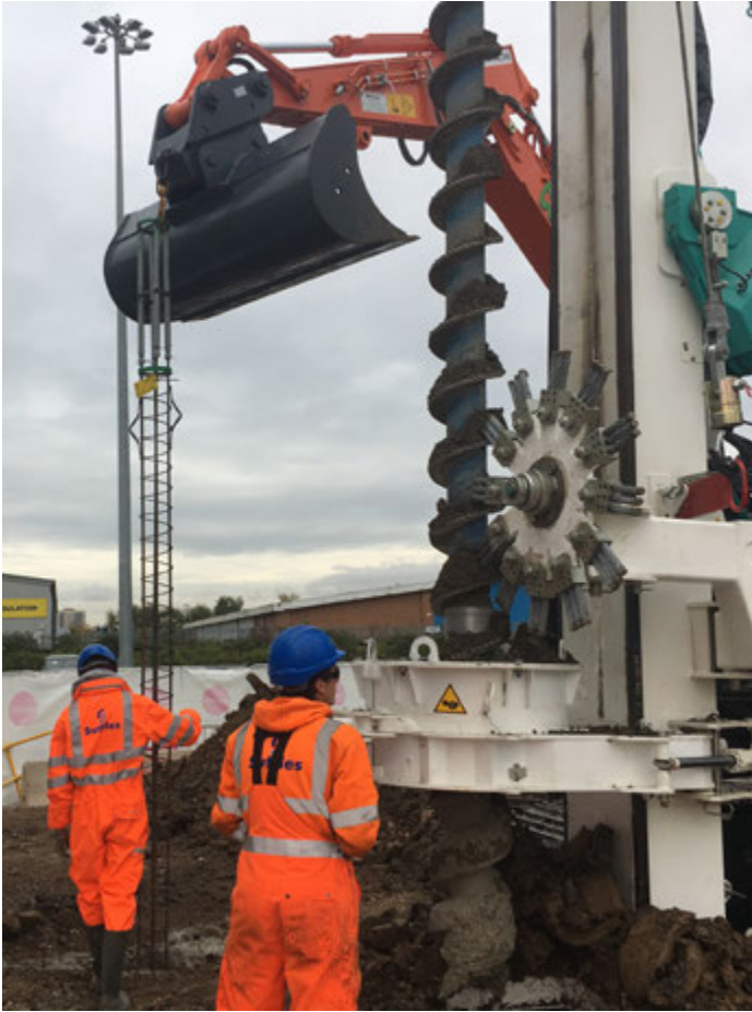
(L-R) A Casagrande B125 was used at Wimbledon Train-care Depot as a deep foundation solution was needed
