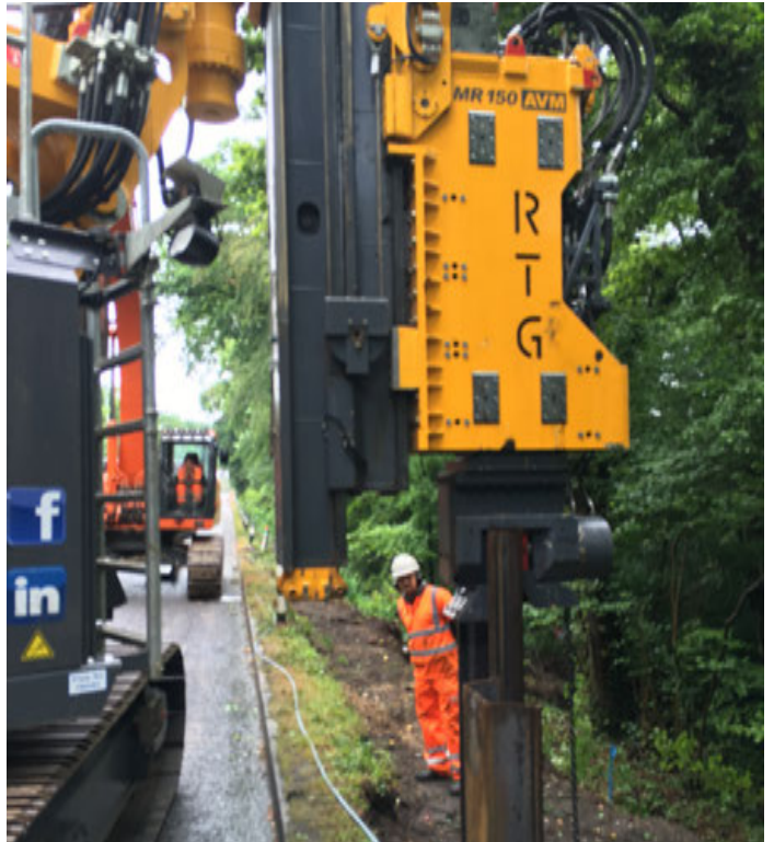
(L-R) An RTG RG16T was used at Gravel Hill, Poole for inserting sheet piling to reinforce the carriageway
