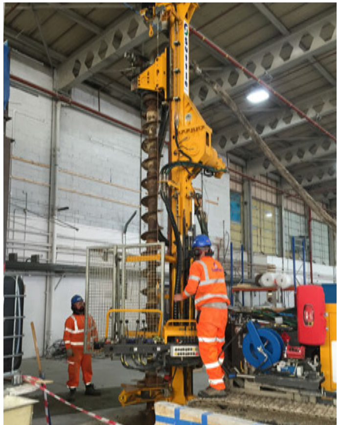
(L-R) A Klemm 708 was used to reinforce the ground for increased loading by a gantry crane at Sunseeker's depot at Osprey Quay, Portland
