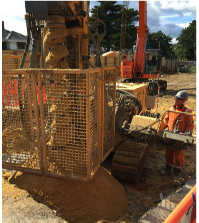
(L-R) A Klemm 709 was used at Canford Cliffs, Poole, to build a retaining wall solution for a basement
