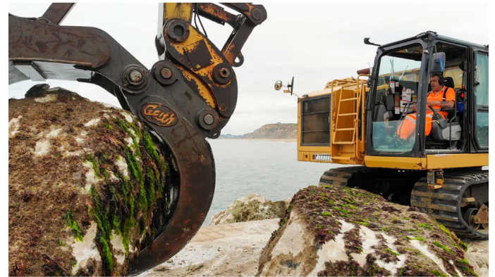
Hengisbury Head Long Groyne from above: (clockwise from top left) the CAT 345 long reach excavator lifting a boulder; the full site; site operative Phil Cork controlling a Morooka MST 2200 tracked dumper; a 48 tonne Volvo excavator
