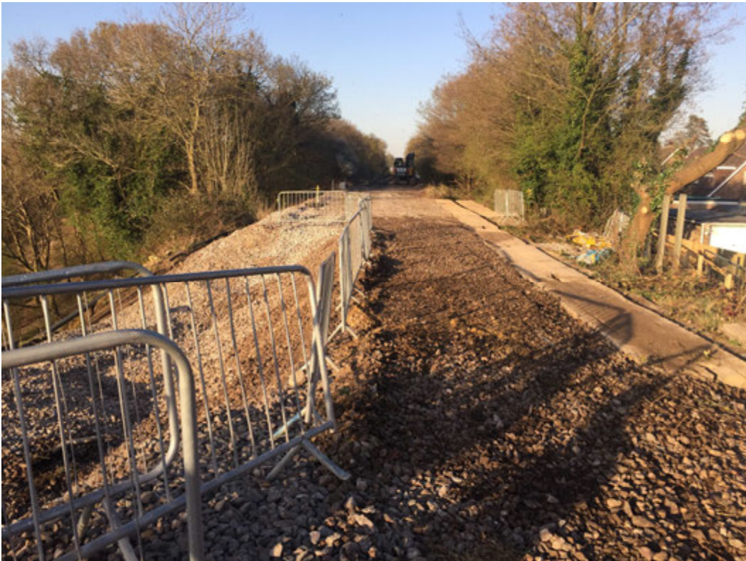
Figure 2: Piling platform at track level
