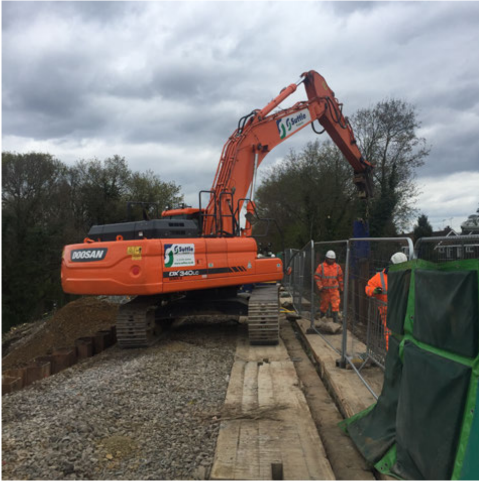
Figure 4: Impact driving at track level
