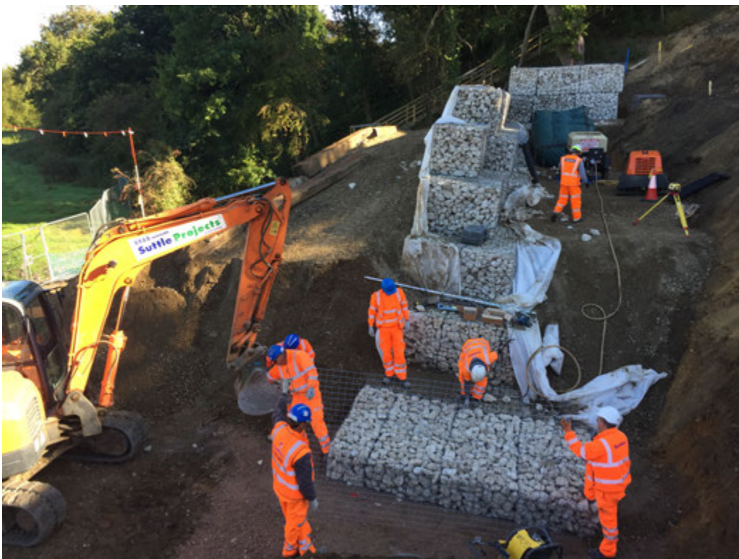
Figure 5: Gabion installation for permanent remediation
