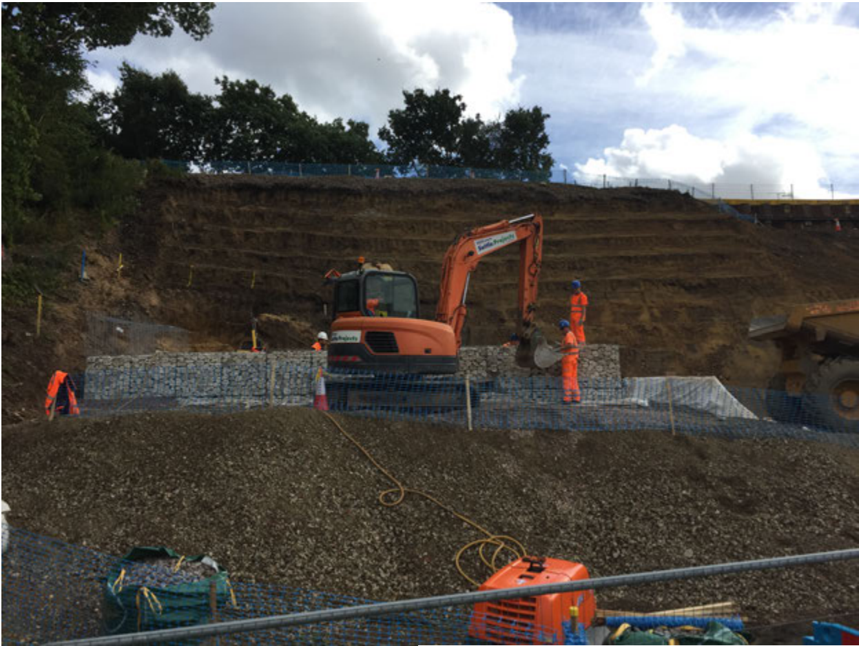
Figure 6: Extensive benching and gabion construction
