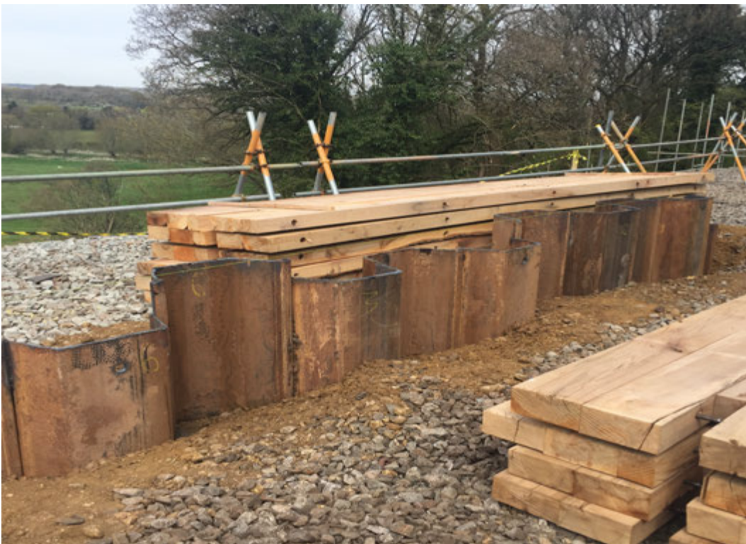
Figure 3: Sheet piles installed in emergency line closure
