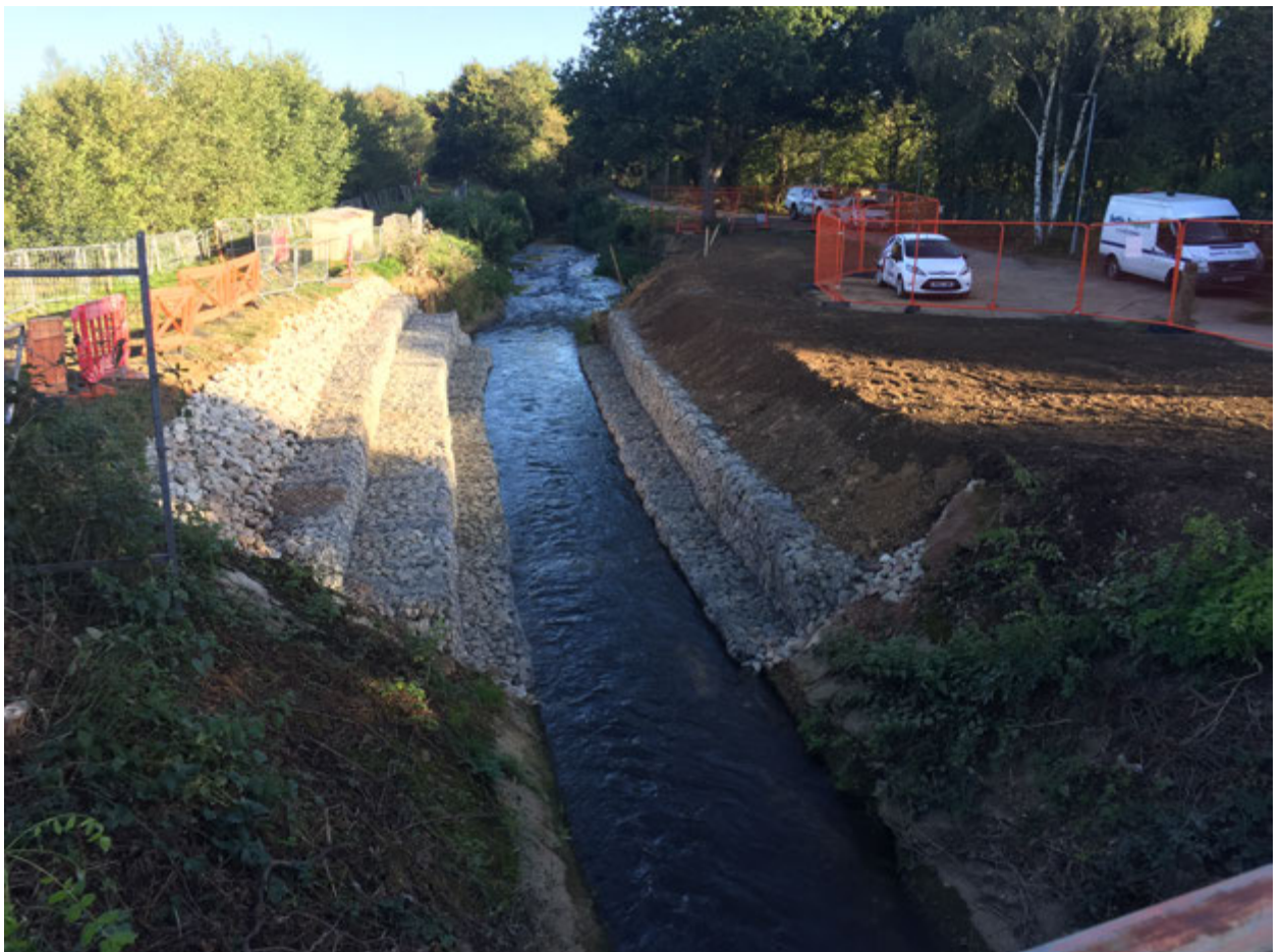
Figure 5: Completed works to channel
