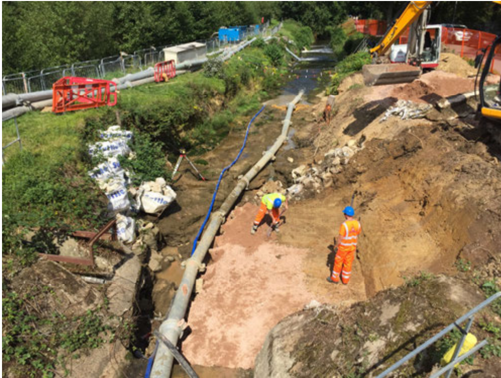
Figure 2: Over pumping in progress with fish pass pipework
