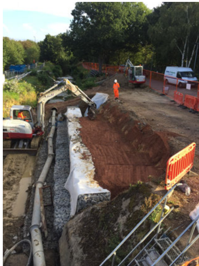
Figure 3: Embankment stabilisation
