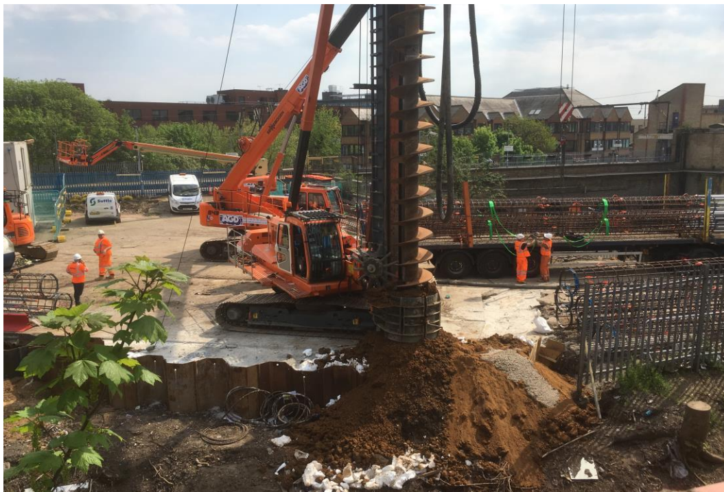
Figure 1: CFA rig supported by a telescopic crane
