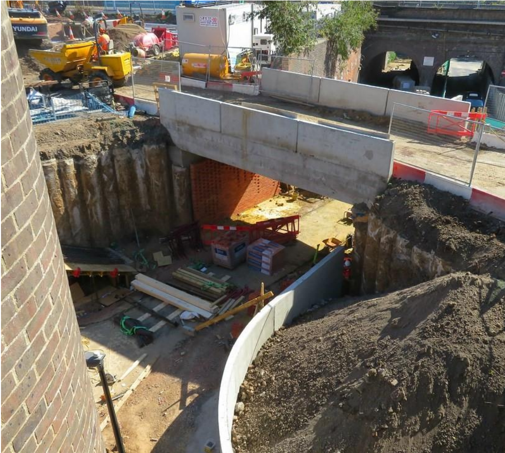
Figure 2: Partial completion of the bridge showing contiguous piles
