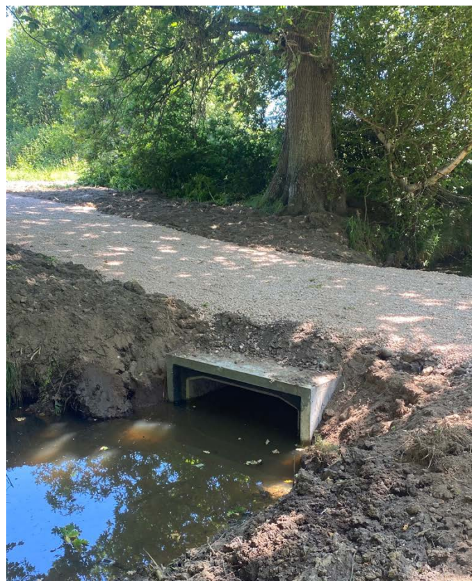
Figure 4: The culvert that was installed
