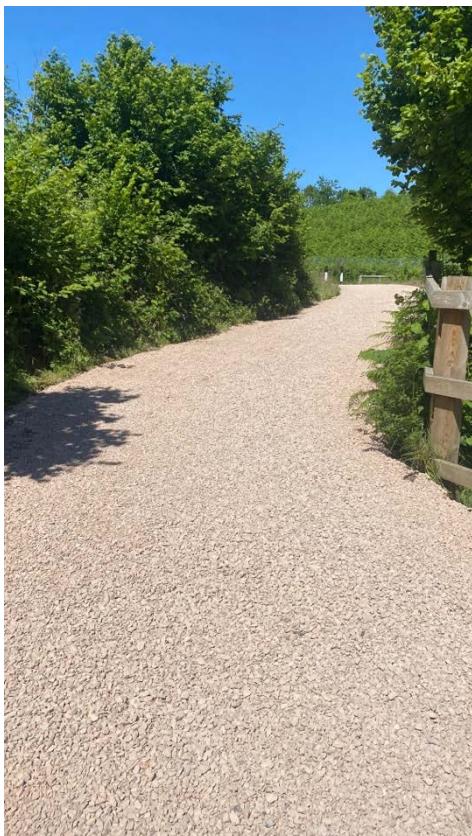
Figure 3: One of the finished paths, topped with chippings
