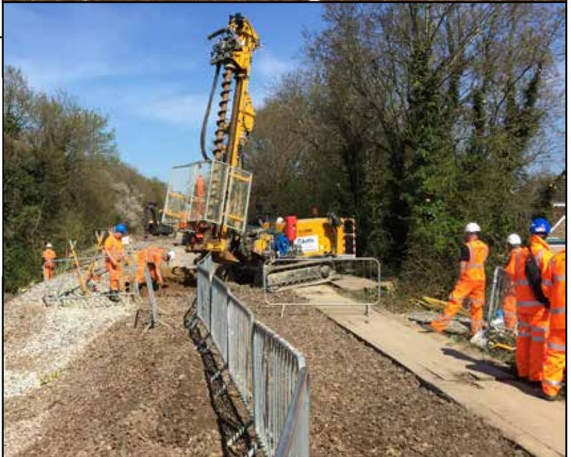
**Ahead of schedule:** a failed railway embankment between Farnham and Alton required pre-drilling and sheet piles
