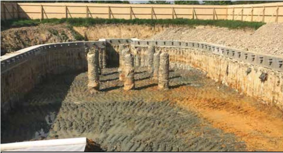
**Breaking new ground:** the secant piling at Woodlands Burial Ground was a first for Suttles
